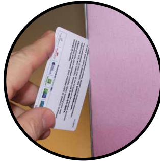
Creates seamless look by using typical credit card along edges
