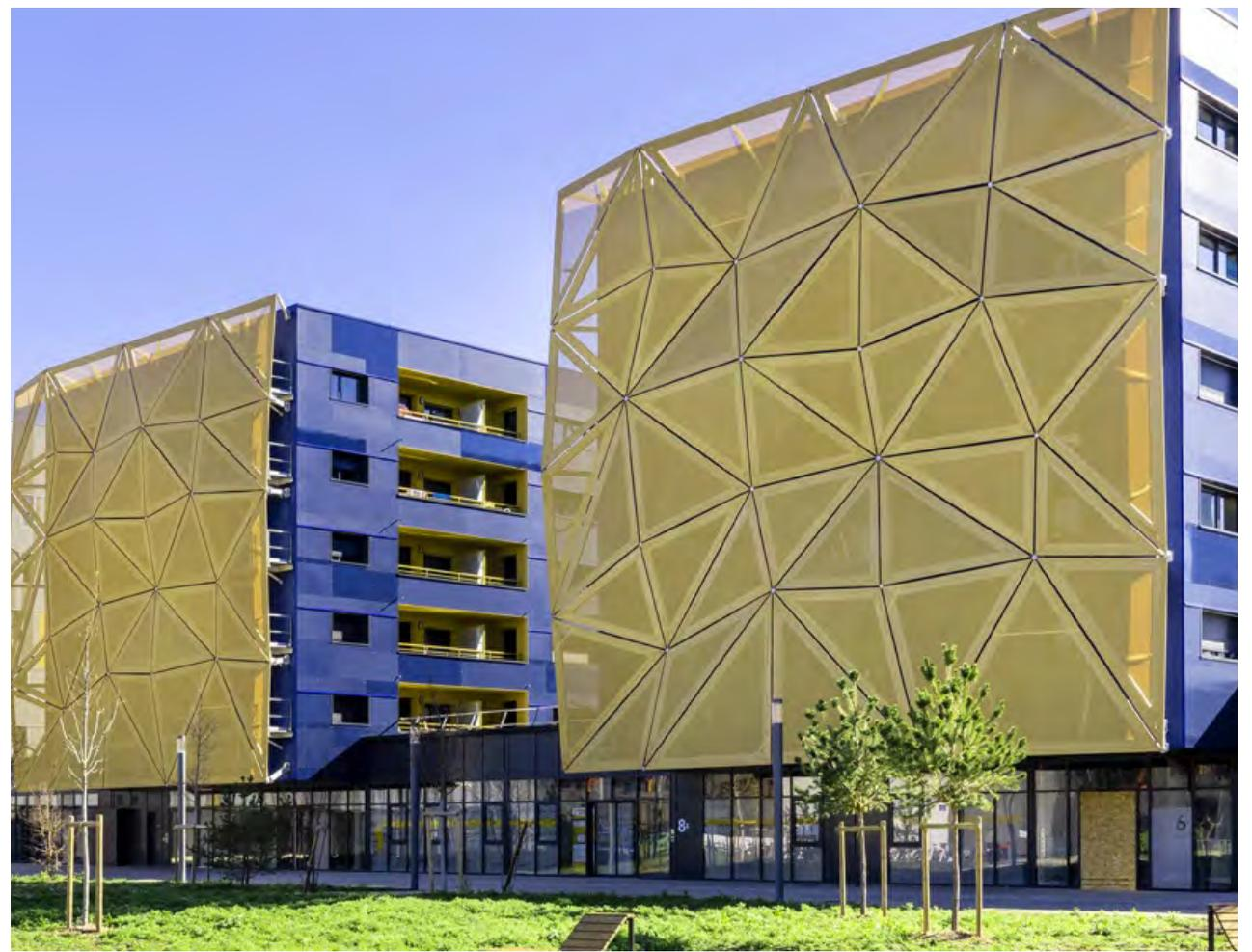
Mesh or vinyl banners are perfectly tensioned using clips in this heavy-duty, large-format banner frame.
