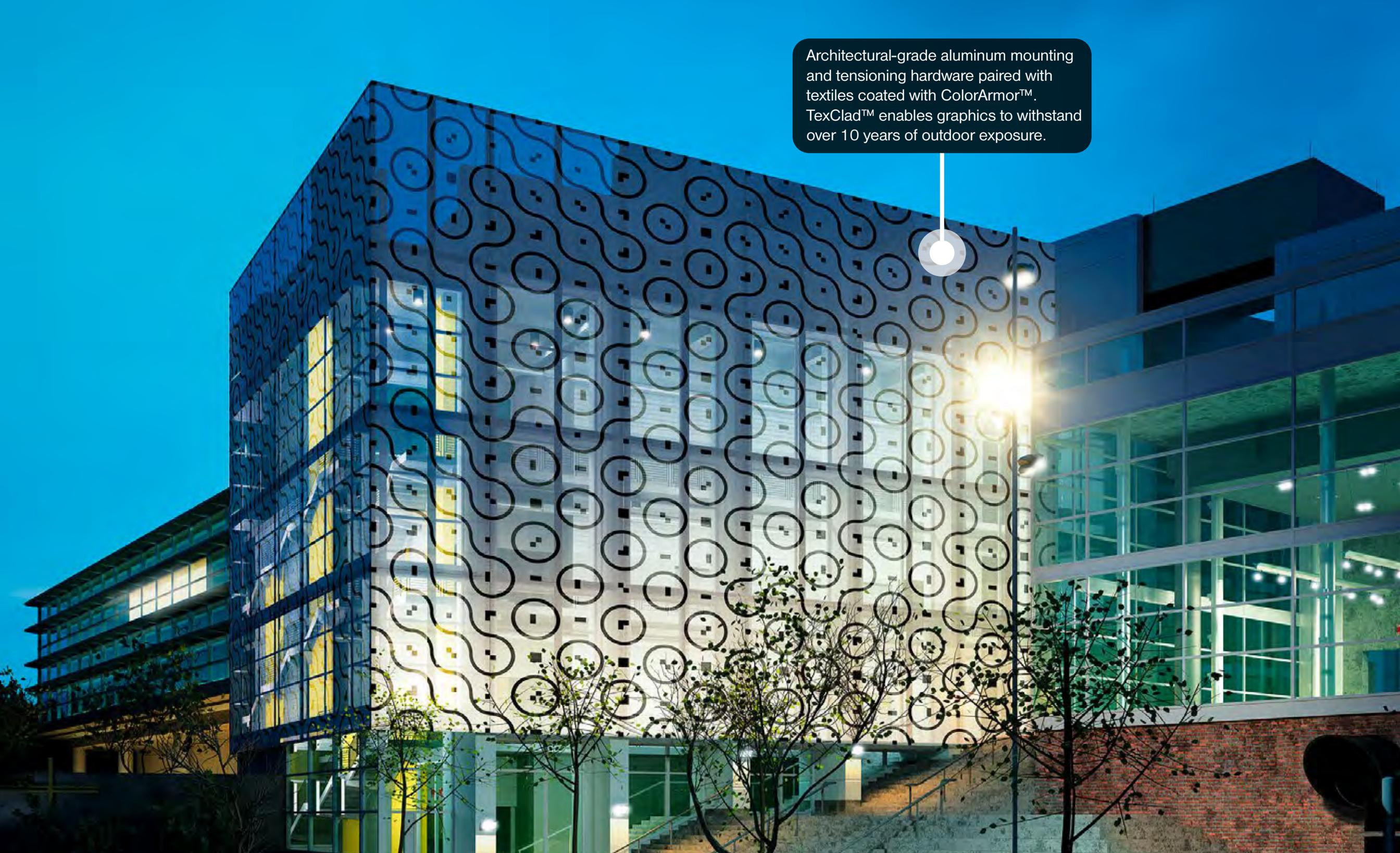
Architectural-grade aluminum mounting and tensioning hardware paired with textiles coated with ColorArmor™. TexClad™ enables graphics to withstand over 10 years of outdoor exposure.
