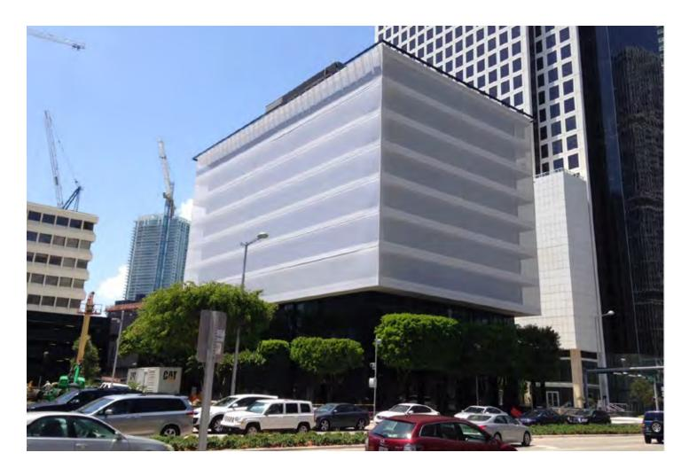
Size: 55,216 sq. ft. of 70% mesh material was fabricated, shipped and installed on all four sides of this seven story building (including over 3,000 linear feet of C-Rail).
